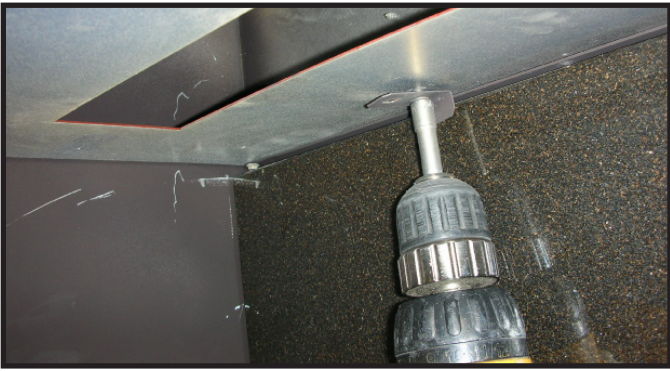
Figure 7. Fastening Angle Tabs to Secure Granite in Place.
